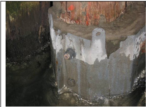
Figure 11. TSA on pile jacket
