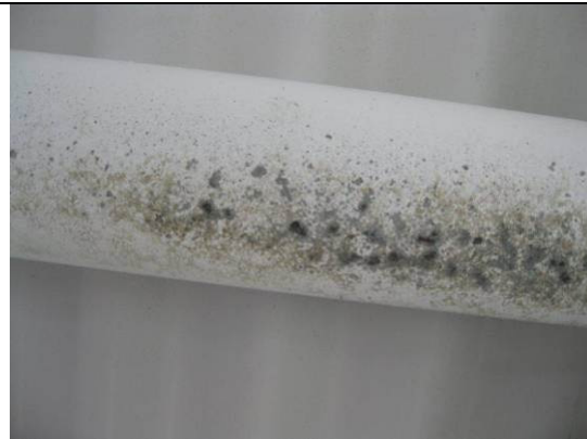
Figure 18. Failure of Duplex TSZ
