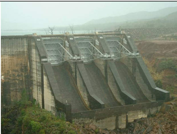
Figure 9. Late Dam gates, New Caledonia
