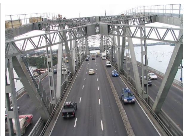
Figure 1. Auckland Harbour Bridge (1958)
